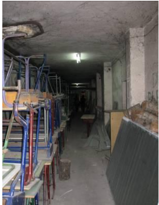
Figure 7. The corridor to the boiler room
